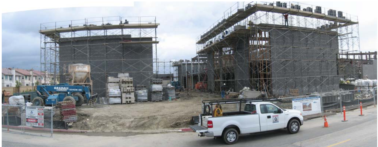
Construction progress as of March 23.
